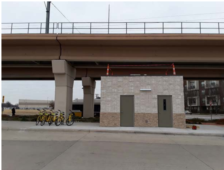
Completed Parkland Medical Station
