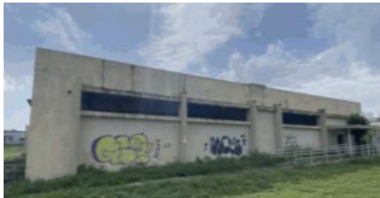
Site; Source: Site Visit
