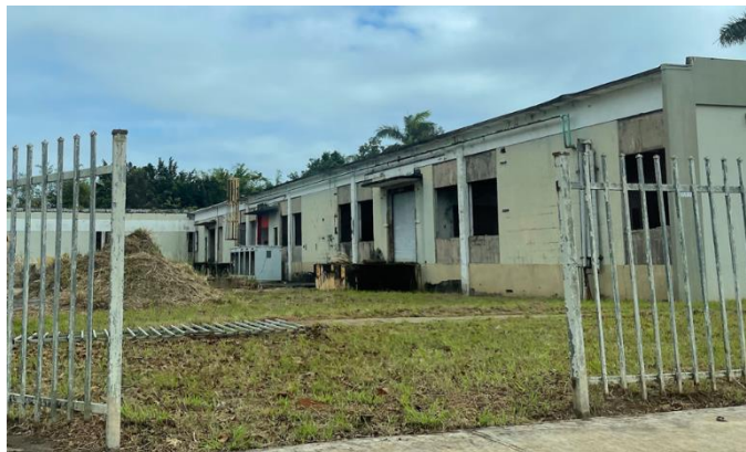
Site; Source: Site Visit
