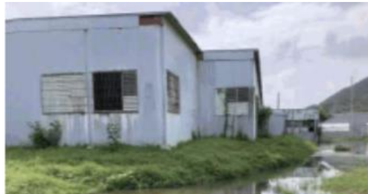
Site; Source: Site Visit
