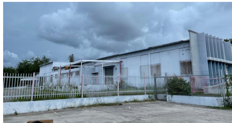
Site; Source: Site Visit
