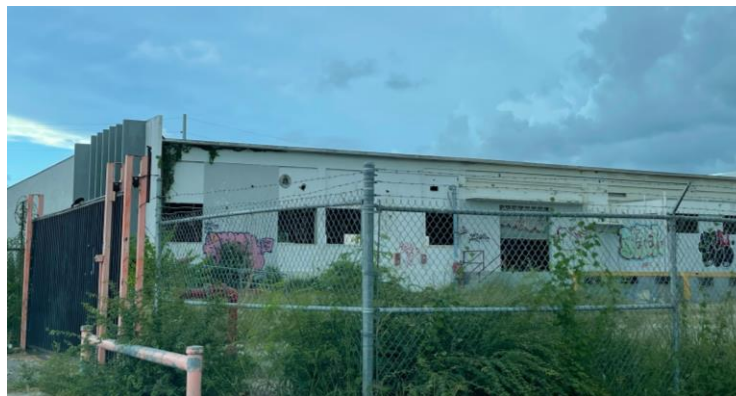
Site; Source: Site Visit
