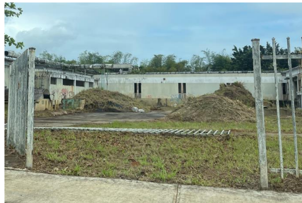
Site; Source: Site Visit
