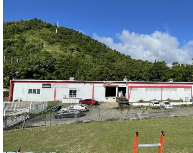
View of the front of building 0951 from road access
