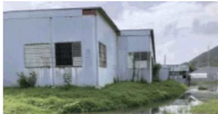
Site; Source: Site Visit
