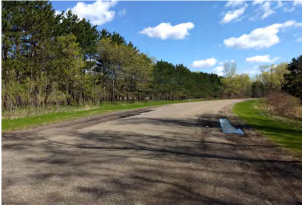
Photo of Existing Roadway
