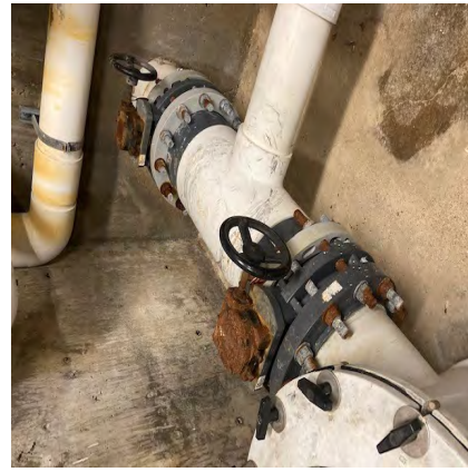
Lazy River Mechanical Room Filtration Replacement. Scheduled for 2026.
