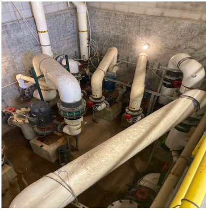
Adventure/Plunge Pool Filtration & Valve Replacement. Scheduled for 2025.
