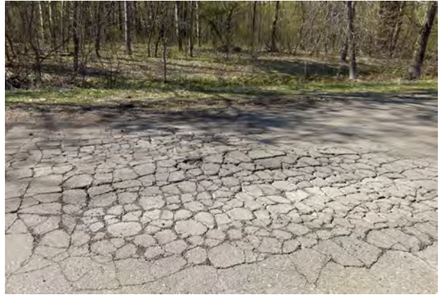
Photo of Existing Roadway
