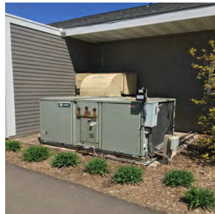
Replacement and upgrade of both Clubhouse air conditioning and heating units.
