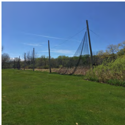
Replacement of the driving range fixtures.
