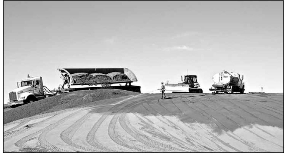
Reconstruction of the Armstrong Blvd./Hwy. 10 interchange in Ramsey is underway.
