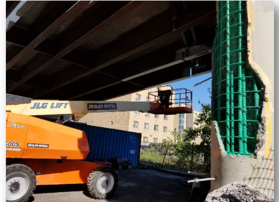
Major Bridge Repair and Rehab
