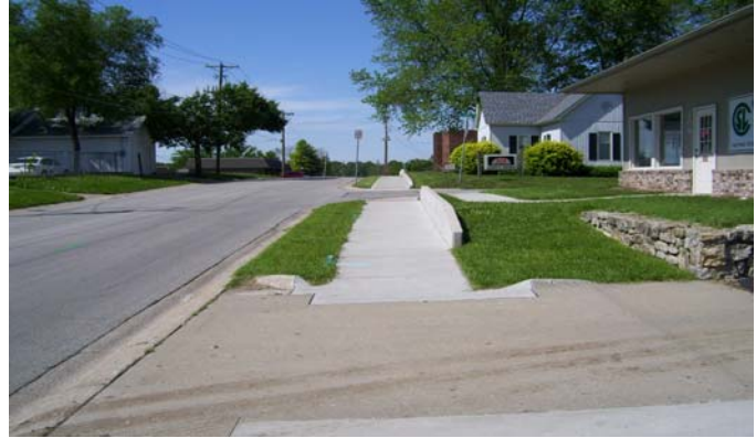
Sidewalk installation (2009-10, CDBG)
