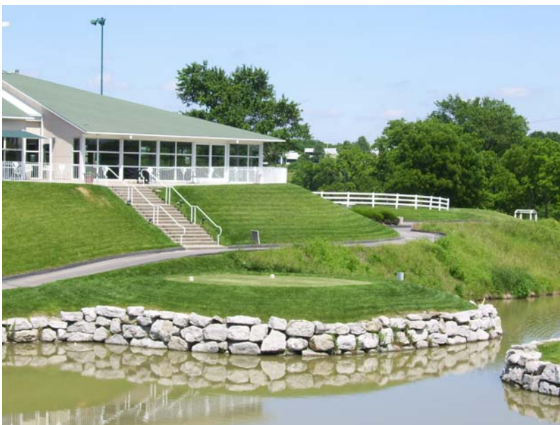
Stone retaining walls at Adams Pointe Golf Course
