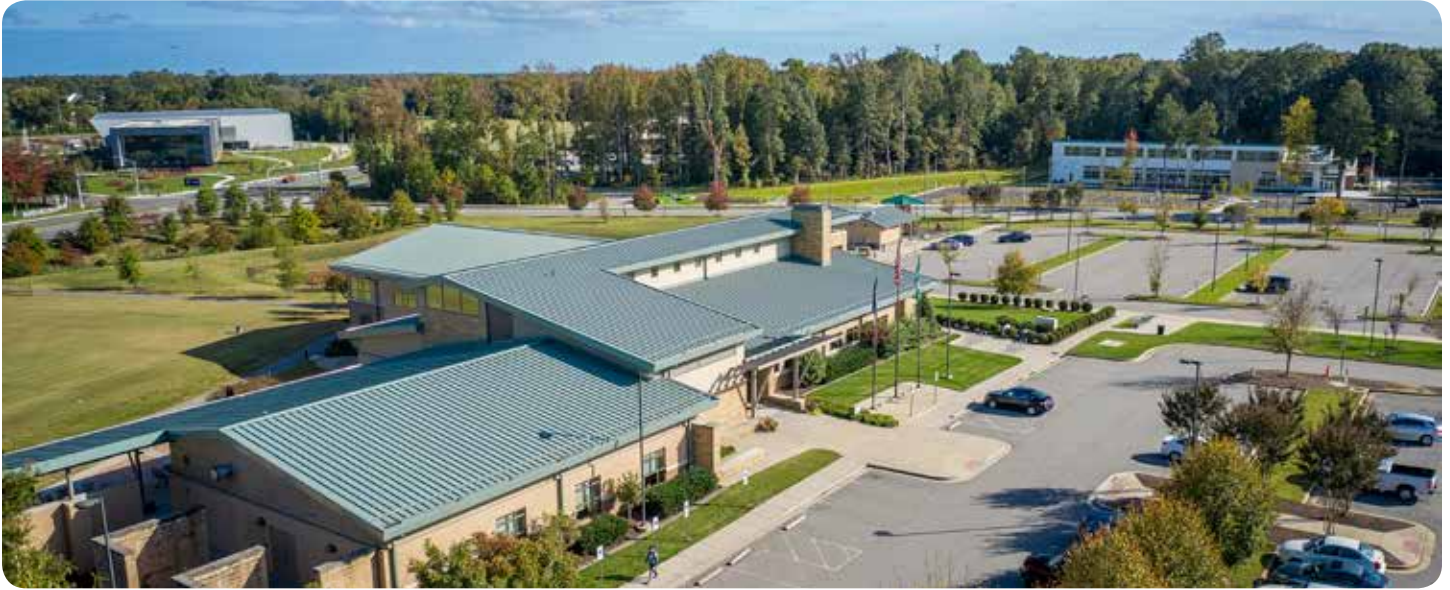
East Laburnum Avenue has seen significant capital investments by the county, including the Fairfield Area Library (upper left), Eastern Henrico Recreation Center (front) and Frank J. Thornton YMCA Aquatic Center (upper right).
