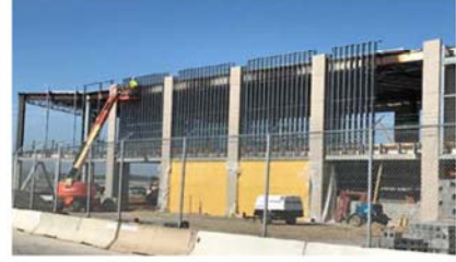
Akron-Canton Regional Airport Authority- Gate Expansion
