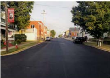
Village of Lewisburg- 2018 Street Resurfacing Program
