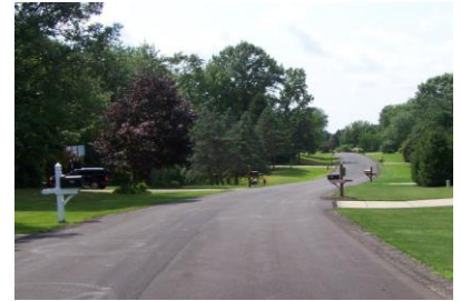
Perry Township Local Road Repaving
