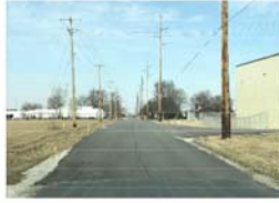
Village of Carey- Roadway Improvements
