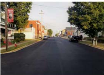
Village of Lewisburg- 2018 Street Resurfacing Program
