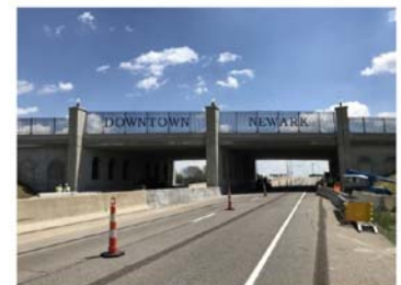
City of Newark - Mount Vernon Road Improvements
