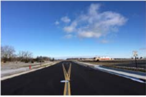
Montgomery County TID- City of Brookville Market Street Extension
