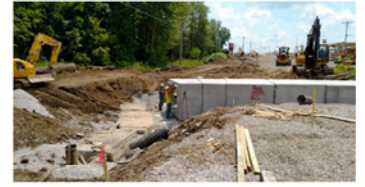
Licking County TID - State Route 310 widening
