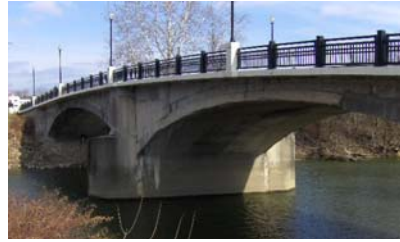
City of Zanesville - State Street Bridge
