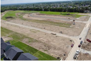
City of Huber Heights Carriage Trails & Windbrooke Public Improvements
