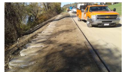
City of Zanesville Wayne Ave (SR60) Improvements
