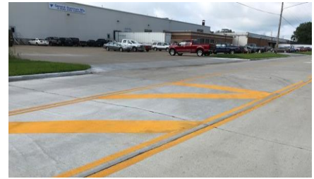
City of Conneaut SR7/SR531 Resurfacing
