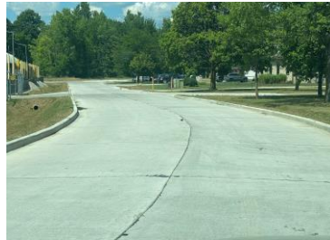
City of Norton Newpark Drive Reconstruction
