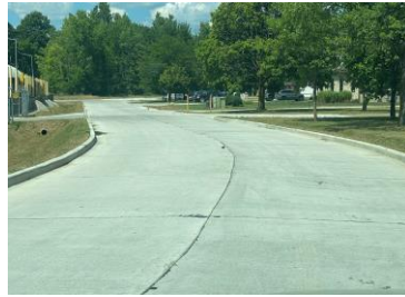
City of Norton Newpark Drive Reconstruction
