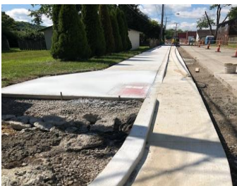
City of Athens Stimson Avenue Improvements
