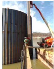
Lawrence County/ KYOVA – Crane Foundation
