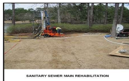
SANITARY SEWER MAIN REHABILITATION
