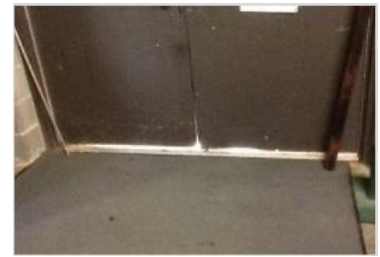
Visible Gap Under Exterior Doors at Holcom Rec Center
