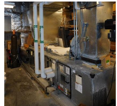
Single Zone Constant Volume Air Handling Unit
