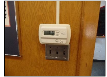
Existing Stand-Alone, Non-Programmable Thermostat
