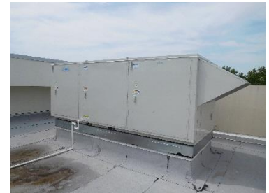
Typical VAV Rooftop Unit
