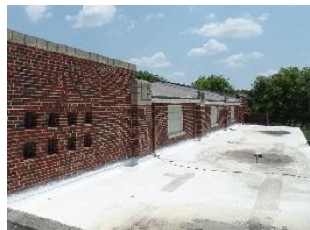
Rubber Membrane Roof
