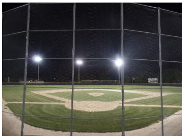
Ice Field with Existing 1500W Metal Halide Lighting
