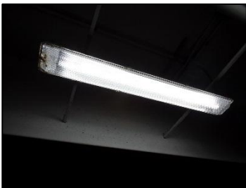
Riverfront garage T5 lighting
