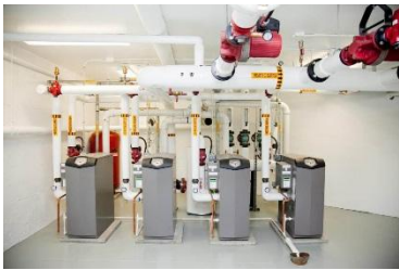
Example High Efficiency Hot Water Plant
