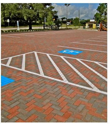
Permeable pavers to minimize stromwater runoff in parking areas, plazas, and streets (source: Gulf Coast Pavers, Inc.)
