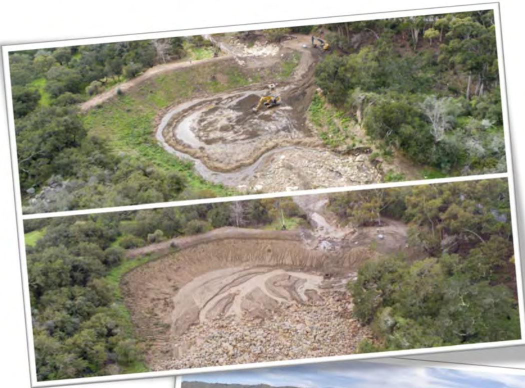
On February 1, 2019, the Romero Canyon debris basin was cleared in anticipation of an approaching storm system. The same view on February 2, 2019 shows the debris captured in the basin.
