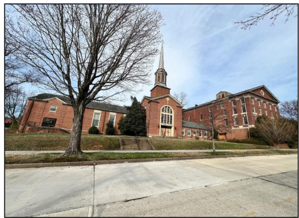
3420 16 th Street NE, Washington DC
