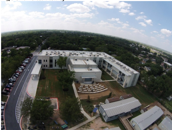
Figure 2: Aerial View of AAM
