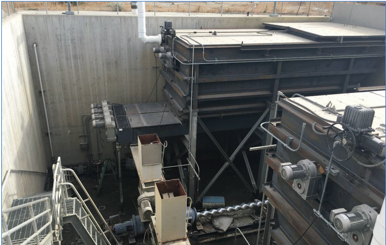
Figure 2-3 Existing Live-Bottom Receiving Bins
