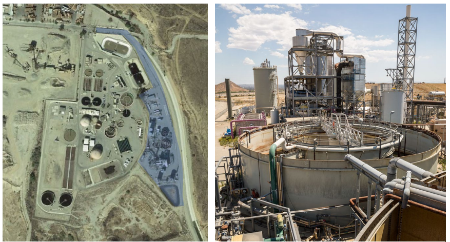
Figure 4: Rialto Bioenergy Facility Site
