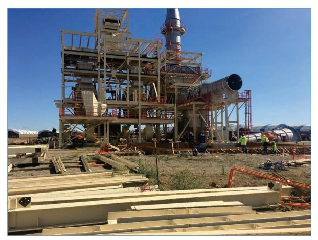
Sifter (left) and Wet Electrostatic Precipitator
