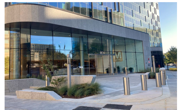
LEED Gold designed facility (Pictured: Metro Headquarters at L'Enfant Plaza)
