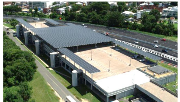
Solar carport installation (Pictured: Anacostia Parking Garage)
