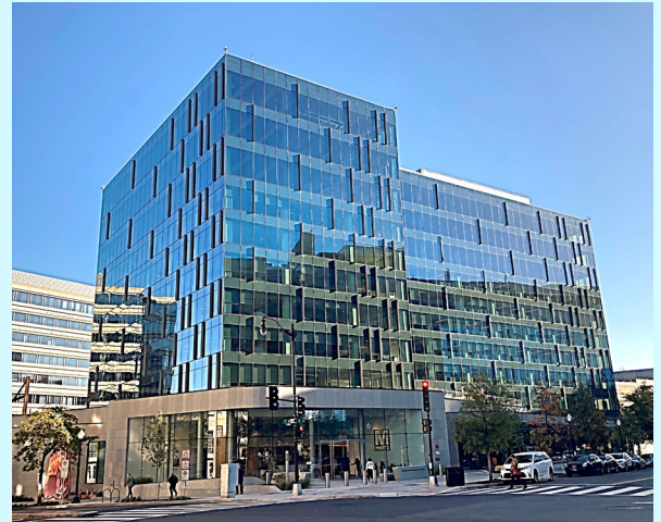
LEED Gold designed facility (Pictured: Metro Headquarters at L'Enfant Plaza)
