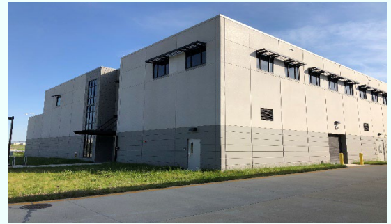
Silver Line Dulles Rail Yard and Maintenance Facility was a collaborative effort between the Metropolitan Washington Airports Authority (MWAA) and Metro (Pictured: Service & Inspection Building at Dulles Rail Yard)
