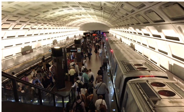
New LED lighting reduces energy use by approx. 60% - each station saves enough to power 40 homes each year.
