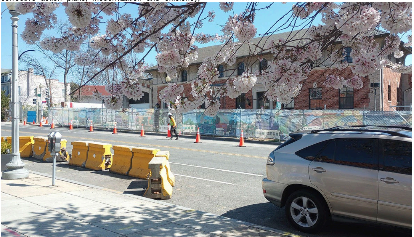
Art in Transit graphic banners around Northern Bus Garage construction
