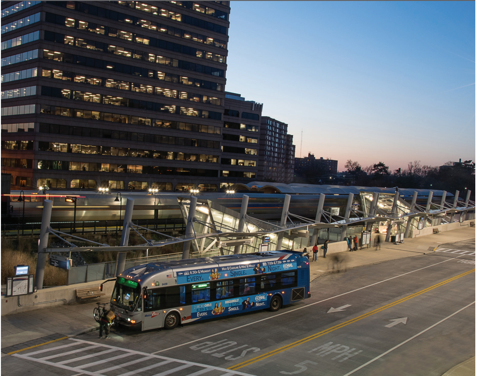
Paul S. Sarbanes Transit Center, Maryland
