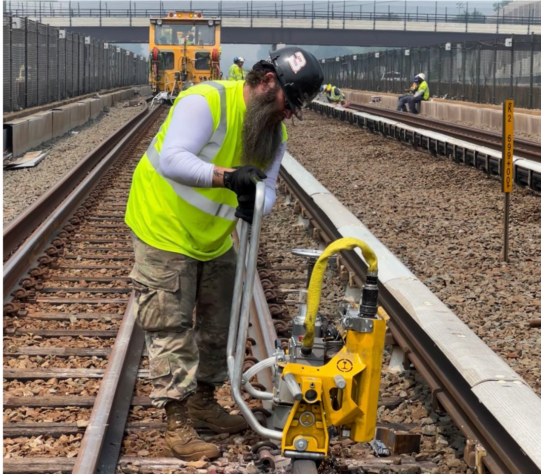
Battery-powered rail surface grinder (K-Line shutdown, summer 2023)
