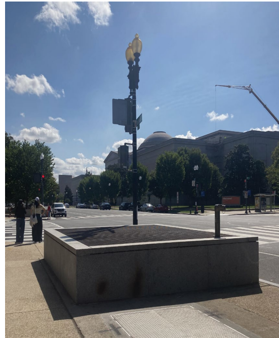
At locations vulnerable to flooding, raised vent shafts can reduce service disruptions (Archives Station)
