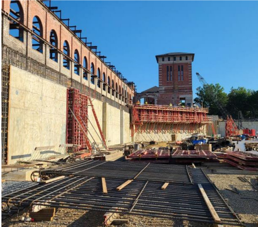
Construction underway at Northern Bus Garage – pursuing LEED®
