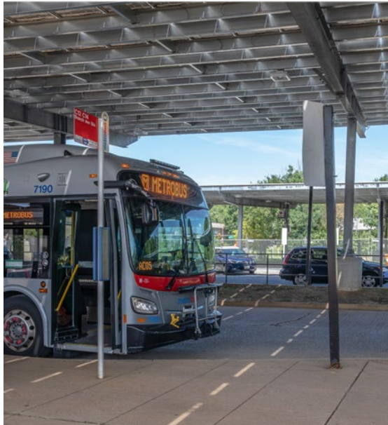
Solar panels at the Naylor Road Station parking lot provide passengers shelter from sun, rain, and snow while waiting for Metrobus
