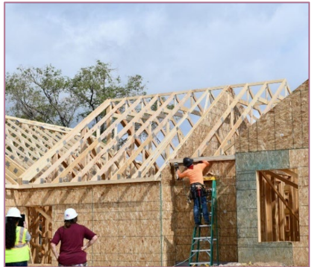
Ramah teacherage homes under construction
