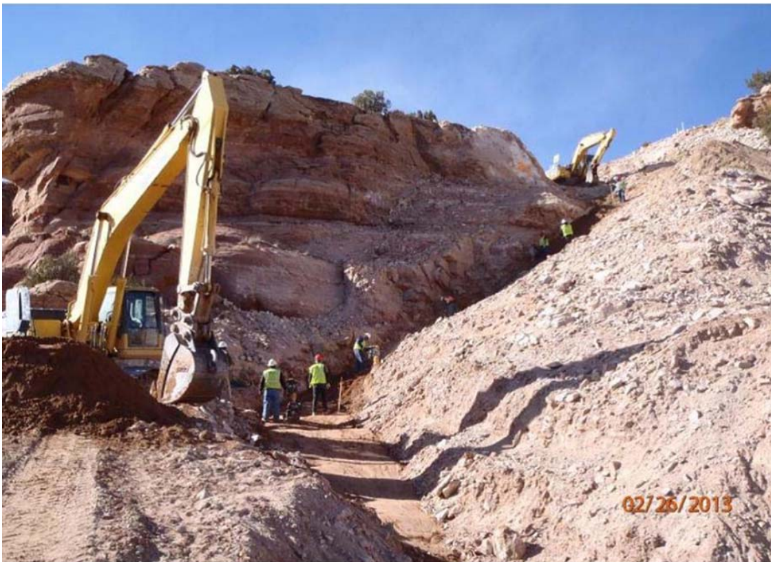
Backfill utilizing bedding material around the HDPE pipe. 12" HDPE WL down the Slope of the Mesa Cliff Worksite WS-21A.
