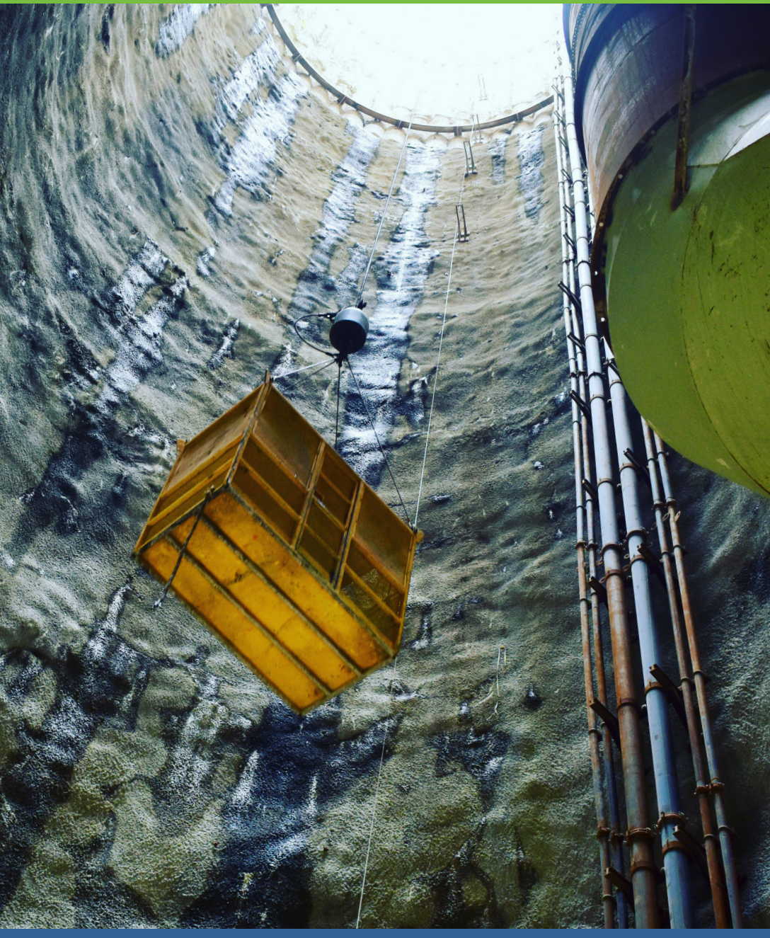
Workers being lowered into MSD's 4-mile Waterway Protection Tunnel. The tunnel will protect the community and our waterways from combined sewer overflows.
