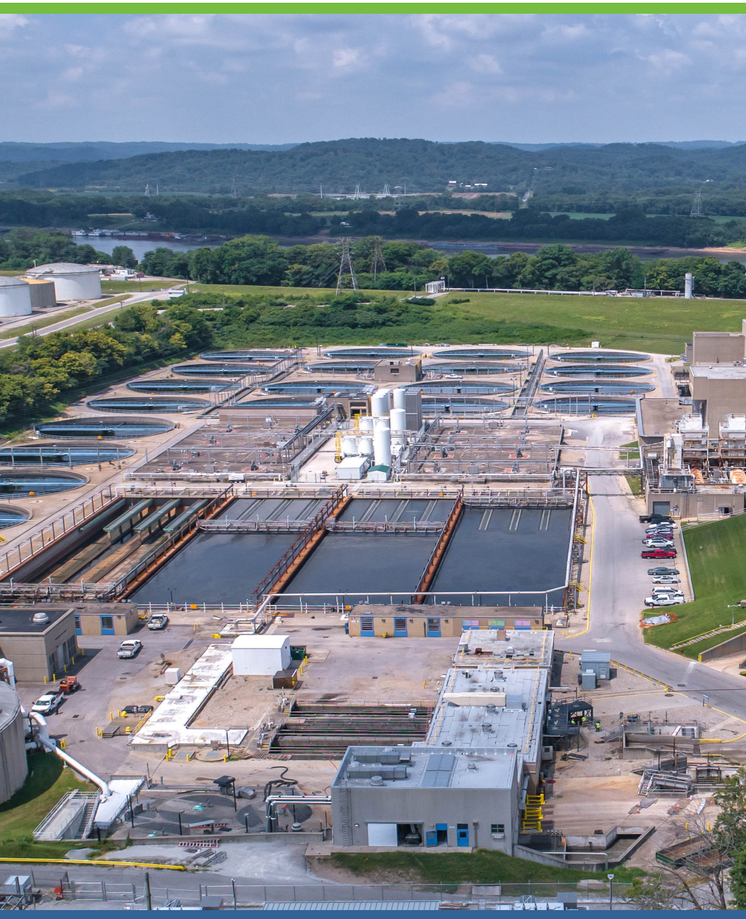
Morris Forman is Kentucky's largest and oldest water quality treatment center. On a normal day, it treats 100 million gallons of wastewater and up to 350 million gallons per day during storms.
