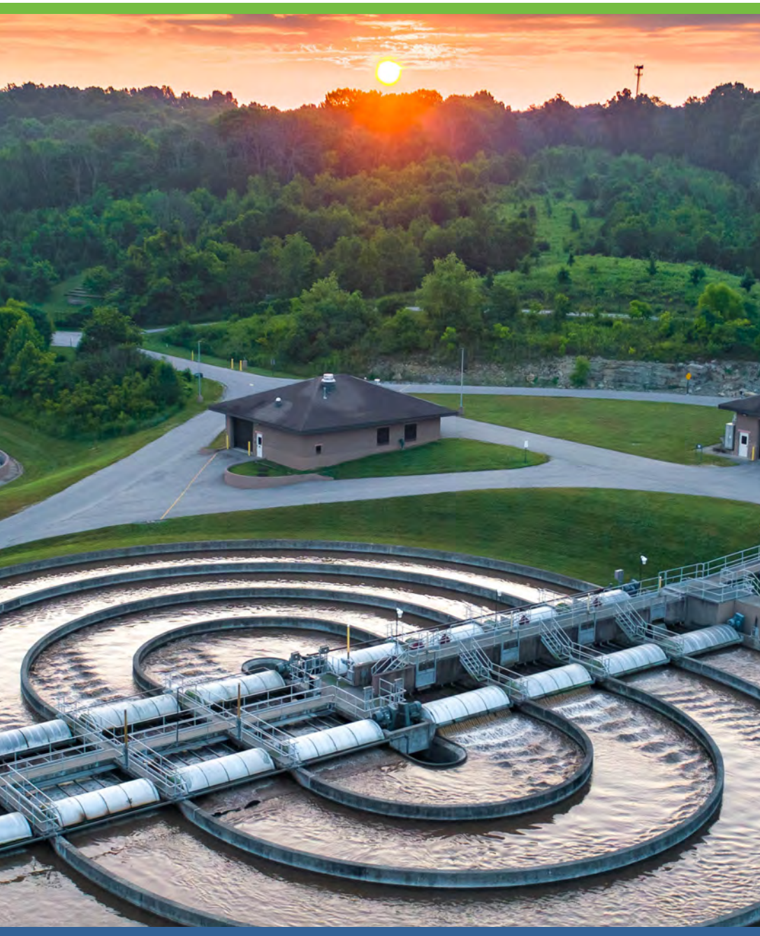
The sun rises over MSD's Floyd's Fork Water Quality Treatment Facility, which is located in Beckley Creek Park.
