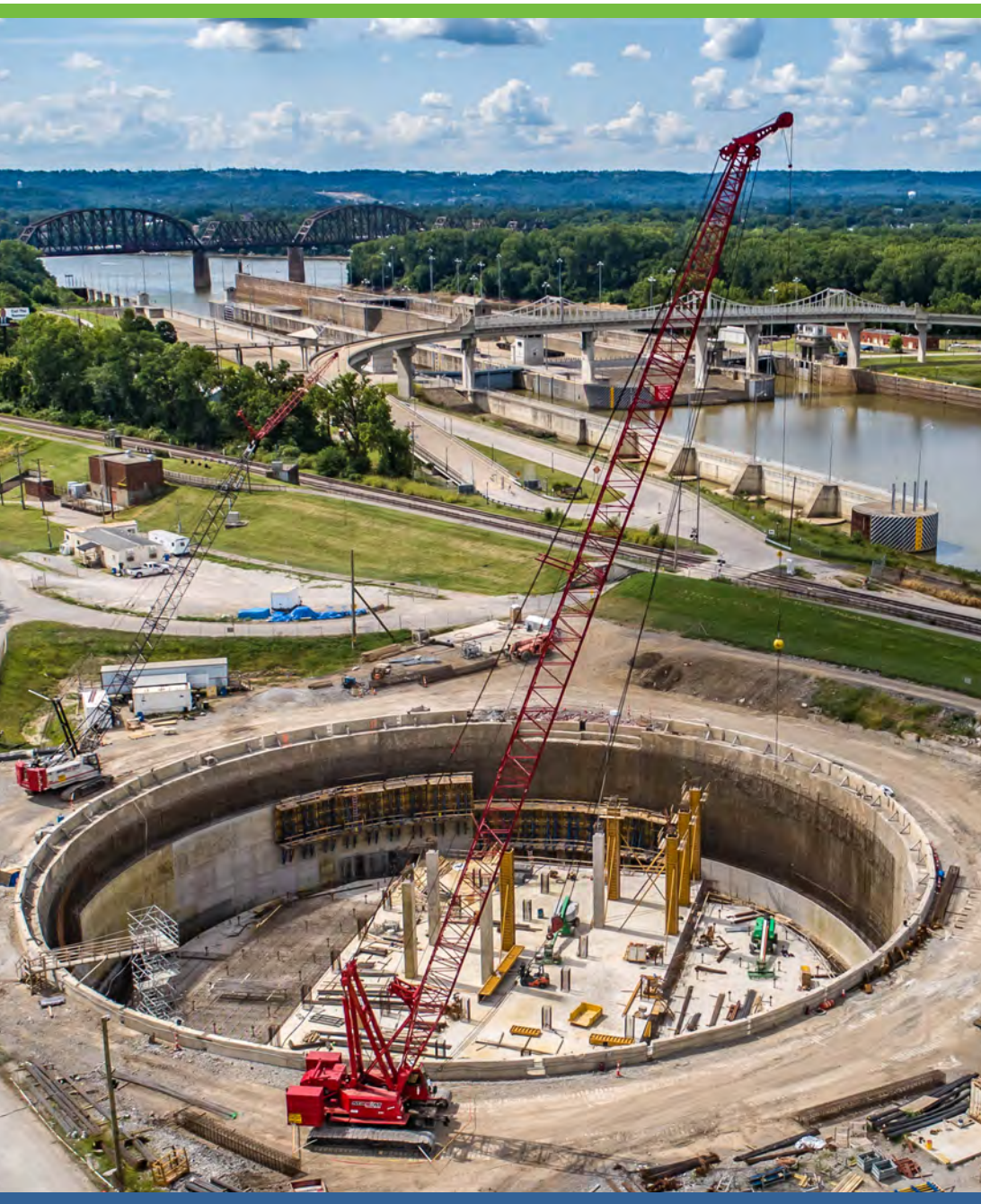
Construction continues on the Portland Combined Sewer Overflow Basin located in Lannan Memorial Park.
