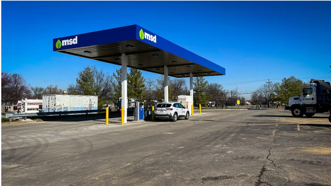
MSD's Central Maintenance Facility
