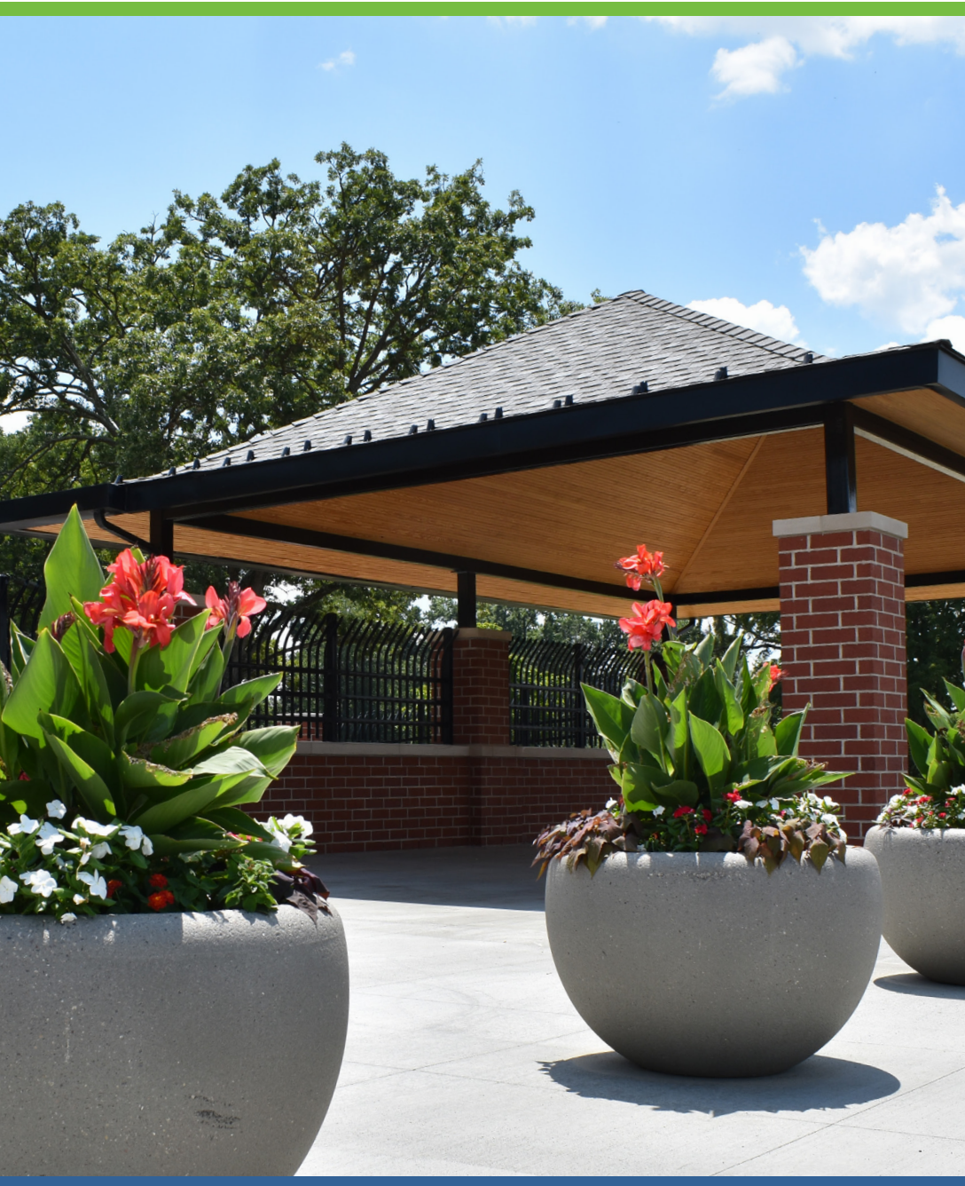
MSD's 20-million-gallon combined sewer overflow basin sits underneath the Great Lawn and this new pavilion, which was a community benefit of the project.
