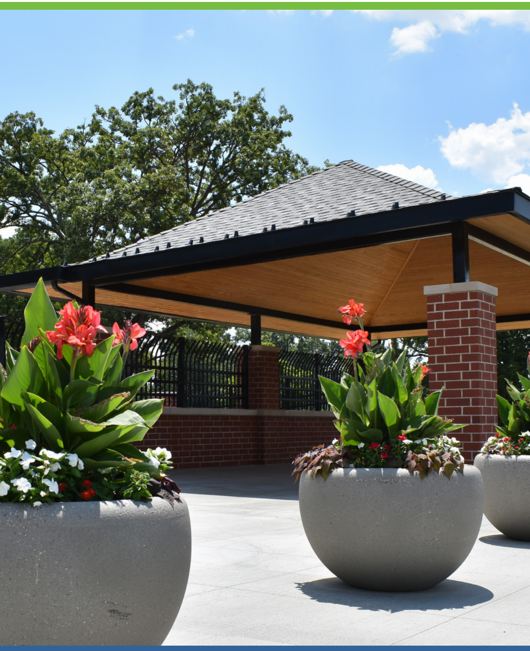
MSD's 20-million-gallon combined sewer overflow basin sits underneath the Great Lawn and this new pavilion, which was a community benefit of the project.
