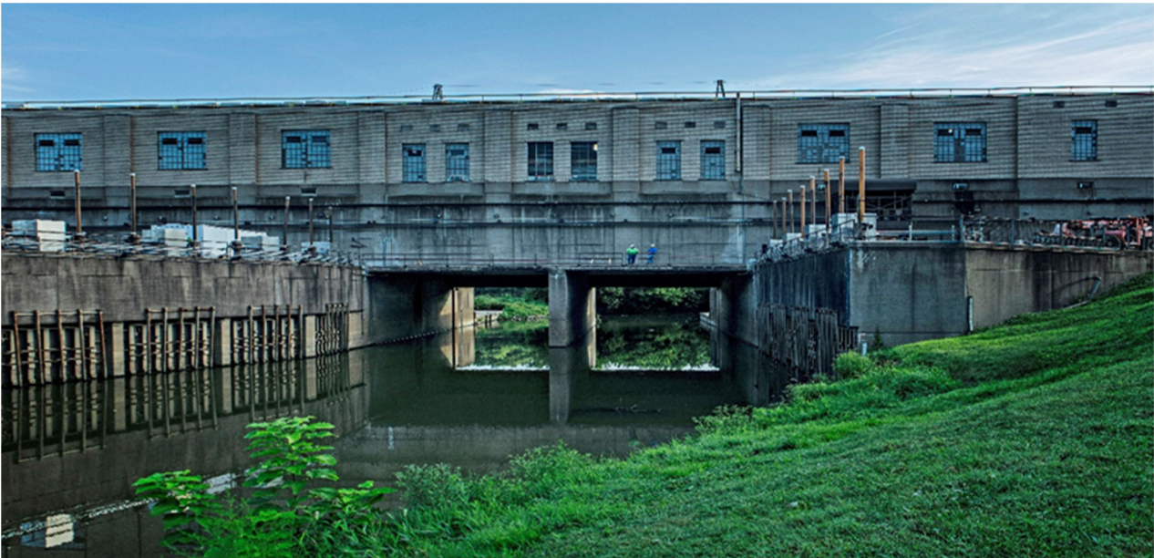
MSD's Beargrass Creek Flood Pump Station.
