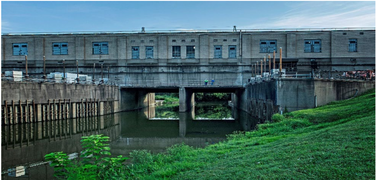
MSD's Beargrass Creek Flood Pump Station.
