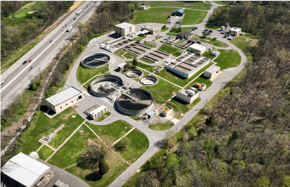
MSD's Hite Creek Water Quality Treatment Center
