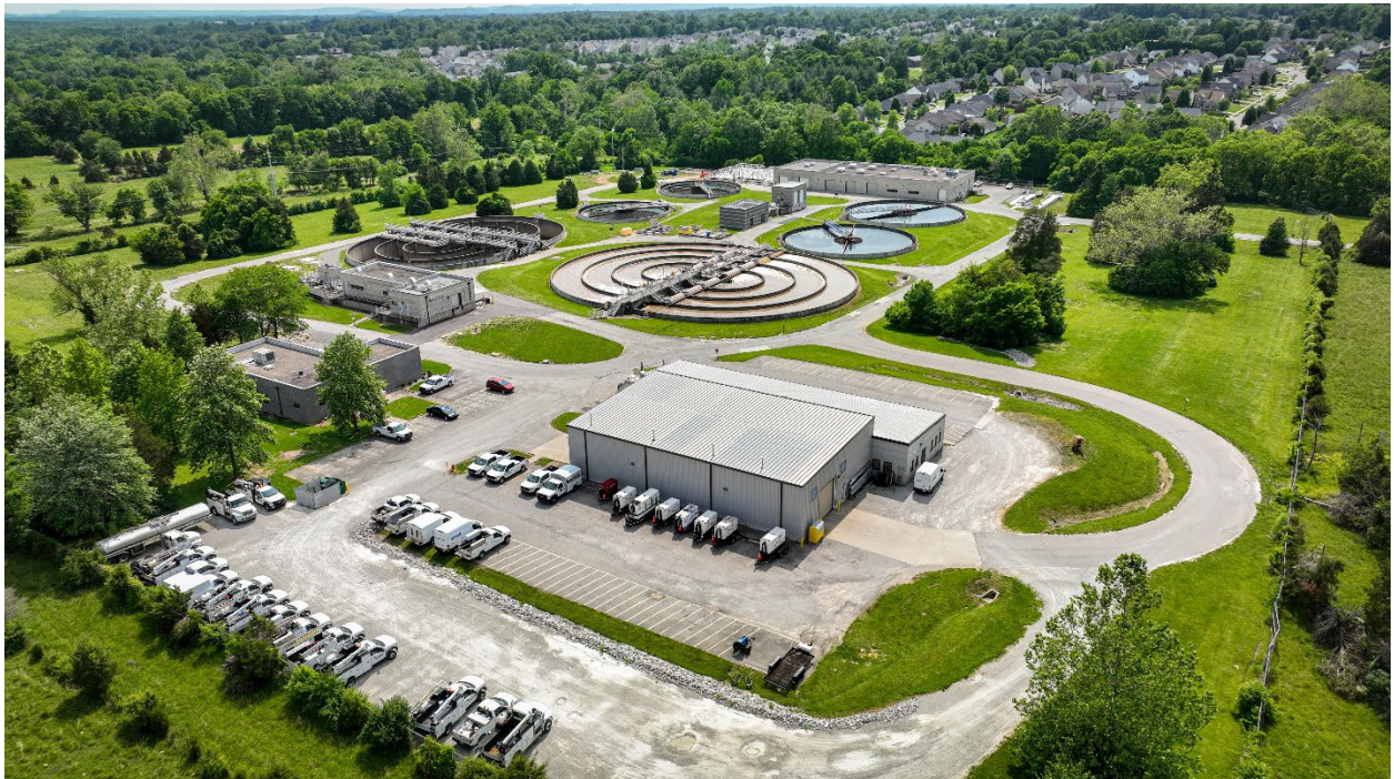
MSD's Cedar Creek Water Quality Treatment Center
