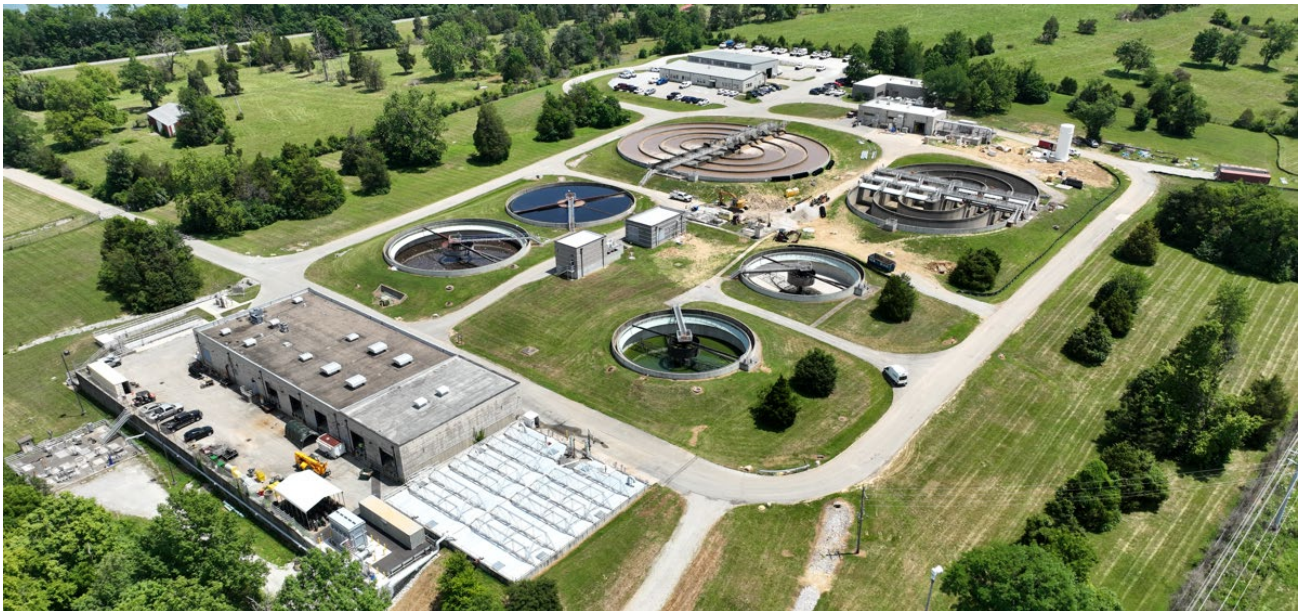
Cedar Creek Water Quality Treatment Center.
