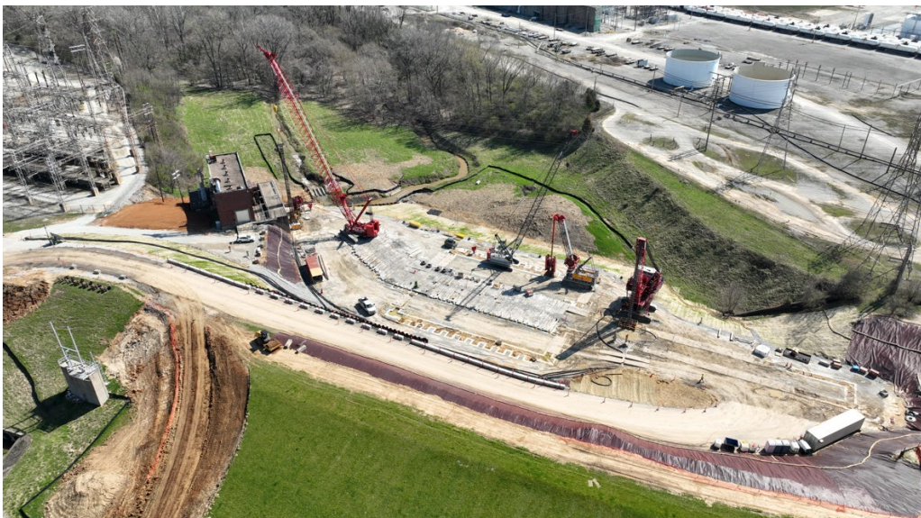
Construction underway at Paddy's Run Flood Pump Station.
