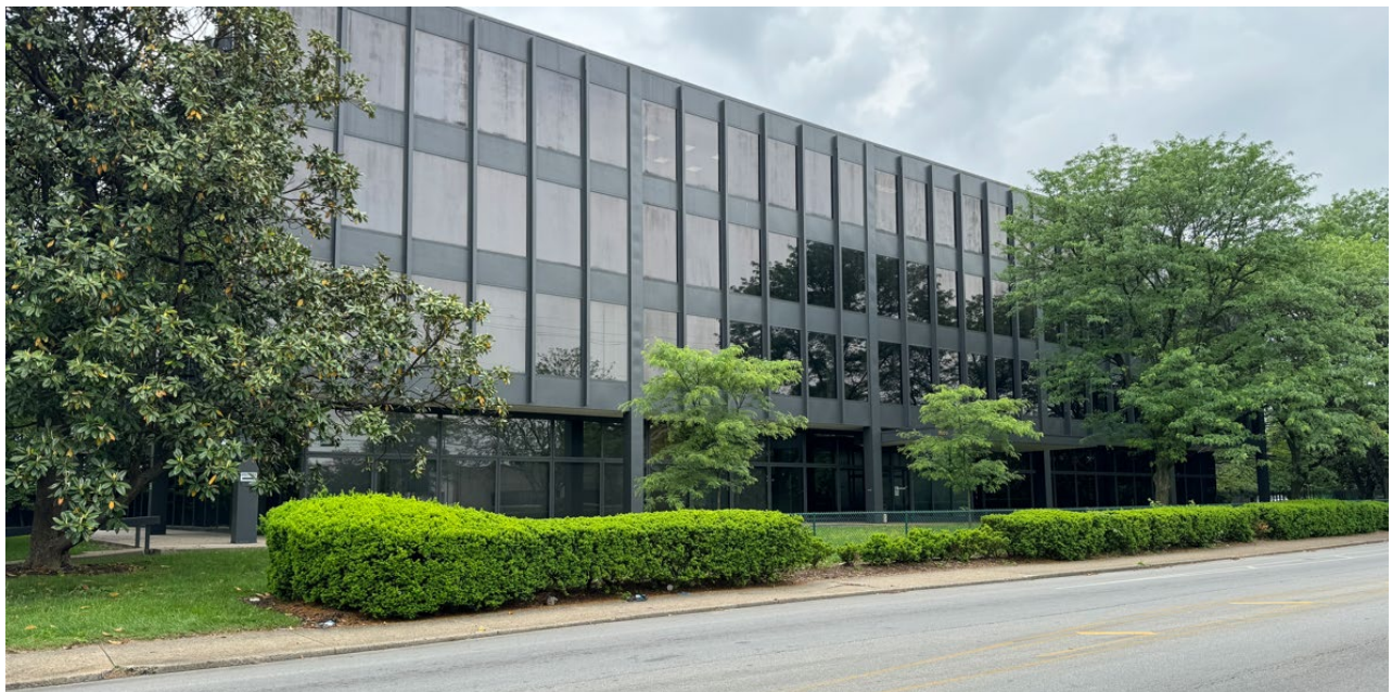
MSD's future Main Office at 15 th & Hill Streets in Louisville's Parkhill Neighborhood.
