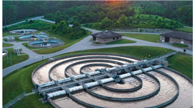
Floyds Fork Water Quality Treatment Center
