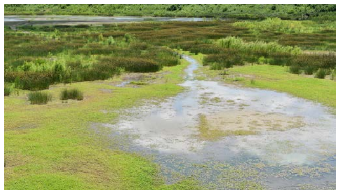
Stormwater Drainage Basin
