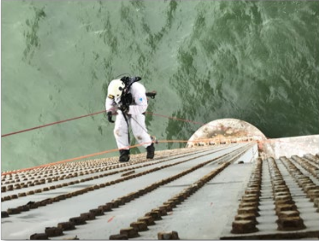
Figure 1-A: Rope access technique to assess details of paint
